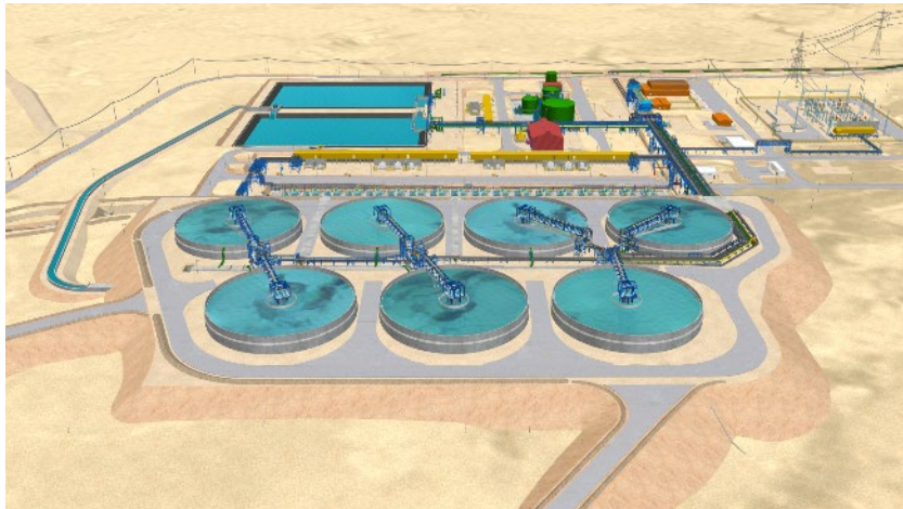
Layout, from the initial request phase in 2023, of the Talabre Thickened Tailings Project (PRET) with the seven DELKOR Thickeners.
