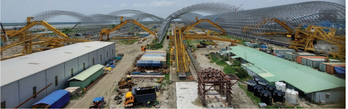
TAKRAF's 6,000tph Rail-mounted Stacker assembled on site in Mexico.
