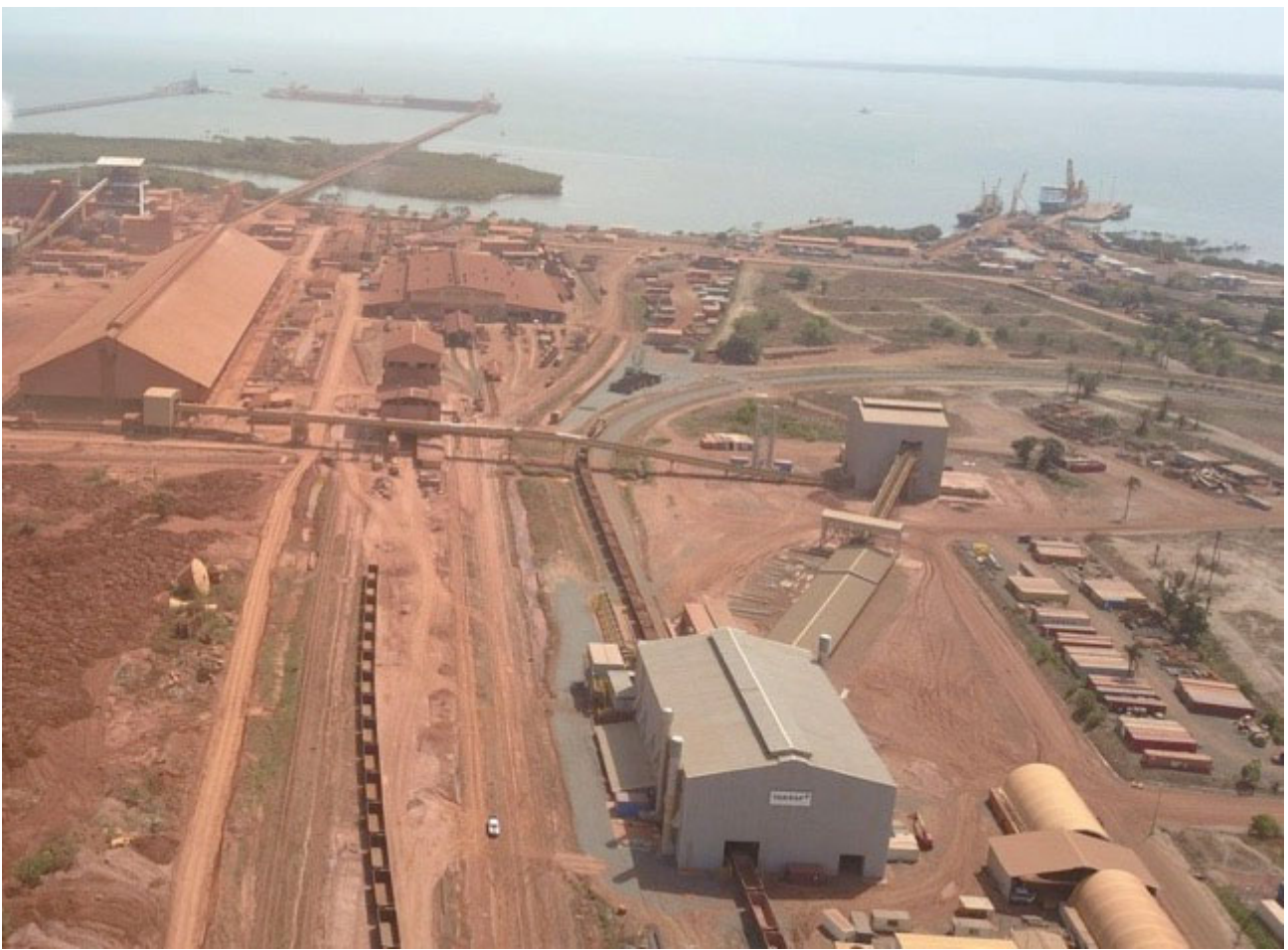
An aerial view of the overall plant in Guinea with the wagon unloading station building from Phase 1 in the foreground.
