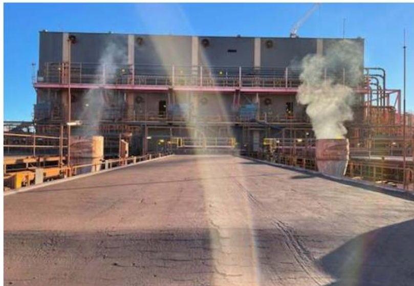
The dramatically improved cake consistency as a result of installing the feeder.
